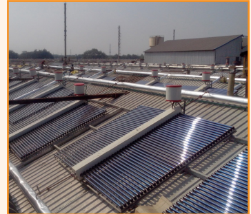
Large Scale Industrial installations
